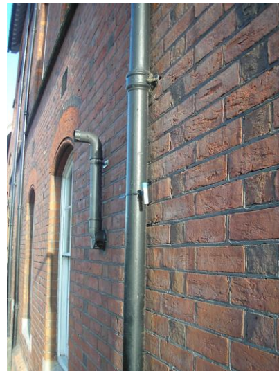
11. North Walls Austen House
